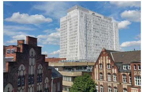
Charité Campus Mitte: View from the campus to the main building after renovation in 2016
